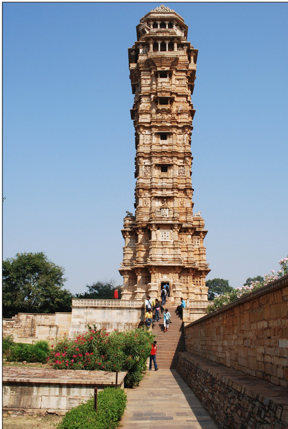
Figure 15: General view of the structural pillar known as VijayStambh, Chittorgarh, Rajasthan.
